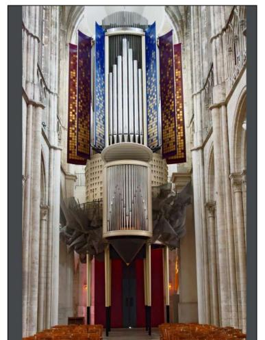
This modern instrument, with its innovative vertical shaped organ case, is perfectly integrated within the Gothic cathedral. The wood and steel structure weighs 20 tons, while the instrument itself weighs only 5 tons. This structure lies on deep foundations which guarantee that it will remain absolutely vertical even if it is completely detached from the stone walls. A very light overhead metal passageway gives access to the console from behind.
